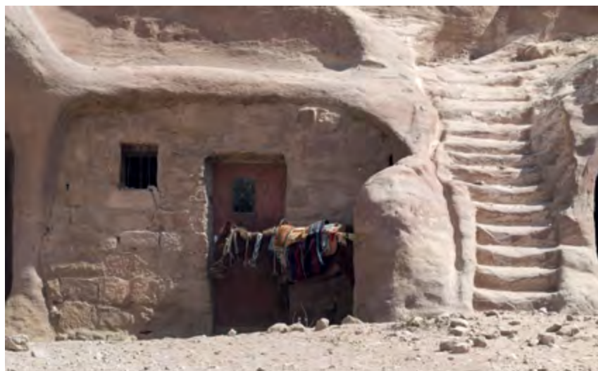
Picture 5. Traditional mudbrick house. After each rain, the house is re-coated with a mixture of clay and chopped straw, which gives the building characteristic smoothed shapes
