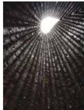
four working days, layer after layer of concrete, each layer 50 cm thick, was poured and rammed around the tentlike structure. In the autumn of 2006, a special smouldering fire was kept burning for three weeks inside the log tent, after which time the tree trunks were dry and could easily be removed from the concrete shell.
